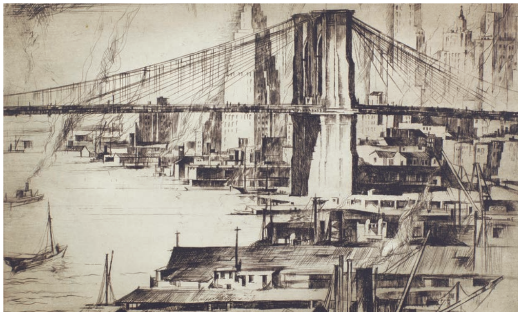
Earl Horter, Bridge Under Construction , ca. 1910. Smithsonian American Art Museum ©
